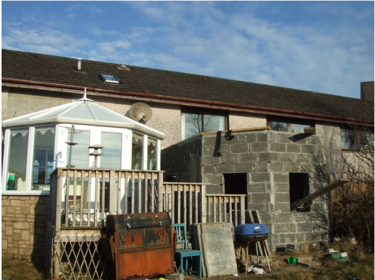
View of conservatory during construction
