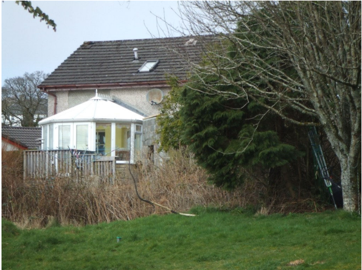
View from Trewince of conservatory during construction
